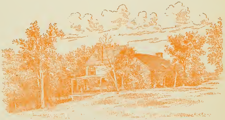
OLD STONE HOUSE AT SOUTH ORANGE.
